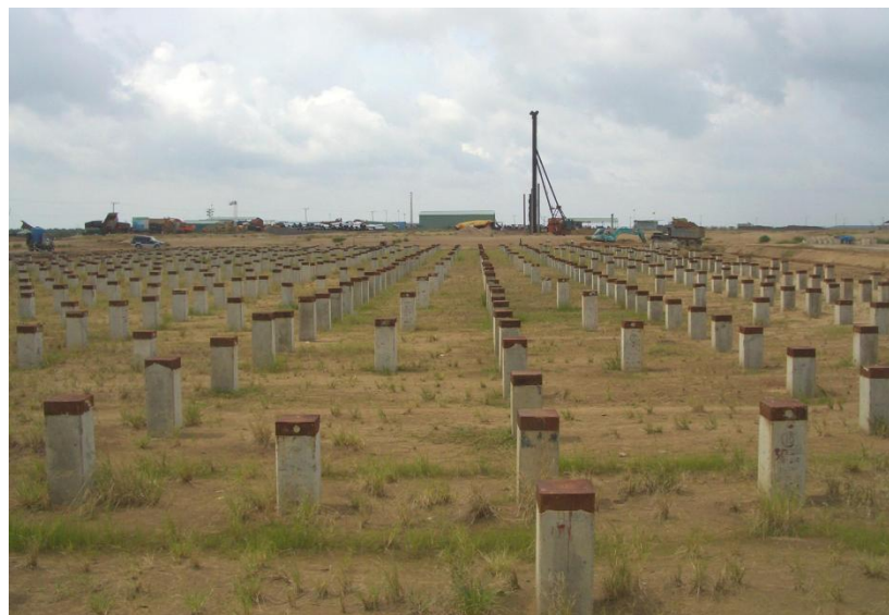
Fig. 14 View on October 4, 2011, from south end of CFS building showing some of the about 750 piles driven for the CFS building. (Authors' photo).
